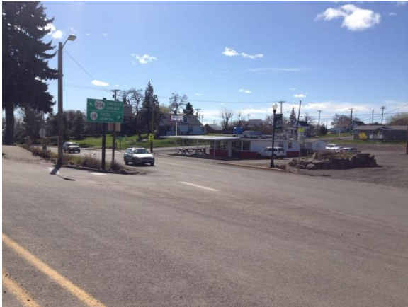
Exhibit 6-1. Restricted Sight Distance at E Bayard Street/Main Street in Condon
