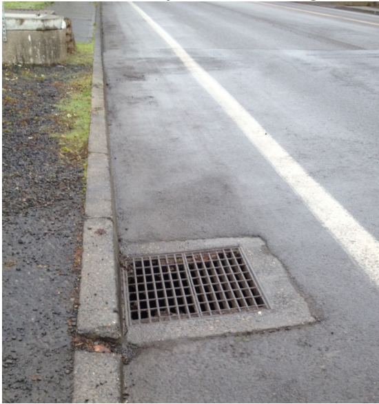
Storm drain grate in the bicycle lane along Main Street (OR47)
