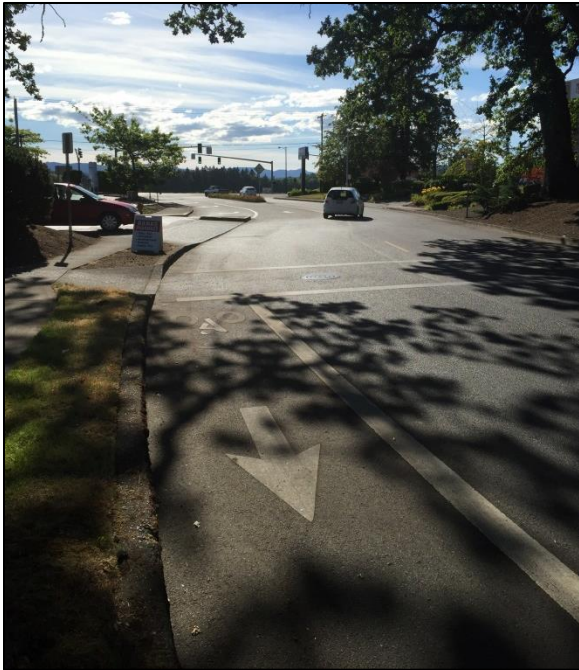
Start of eastbound bicycle lane on NW Oak Way
