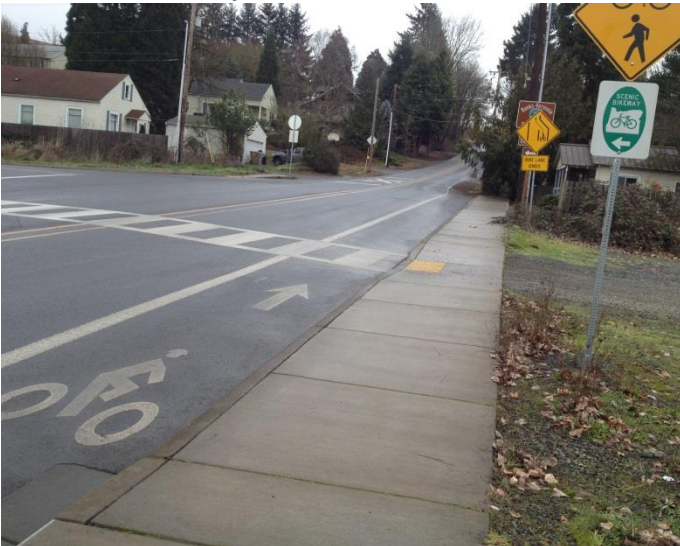
End of eastbound bicycle lane on NW Banks Road
