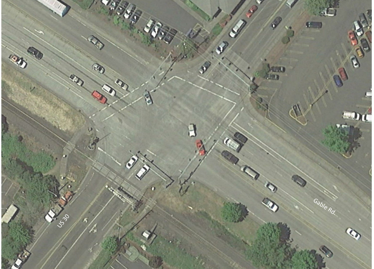
Existing conditions (image: Google Earth)
