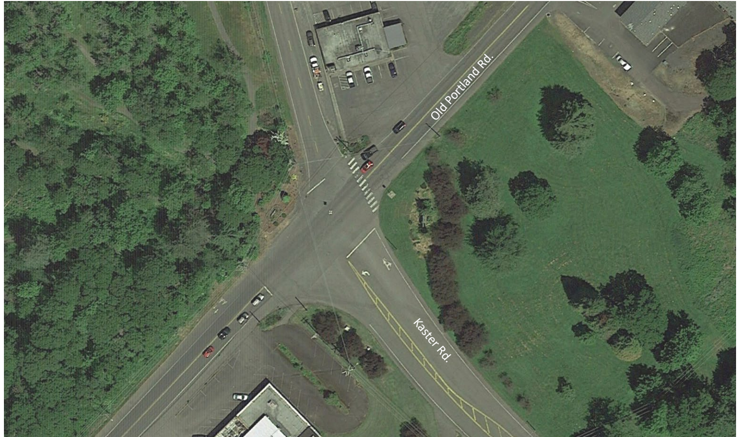
Existing conditions (image: Google Earth)
