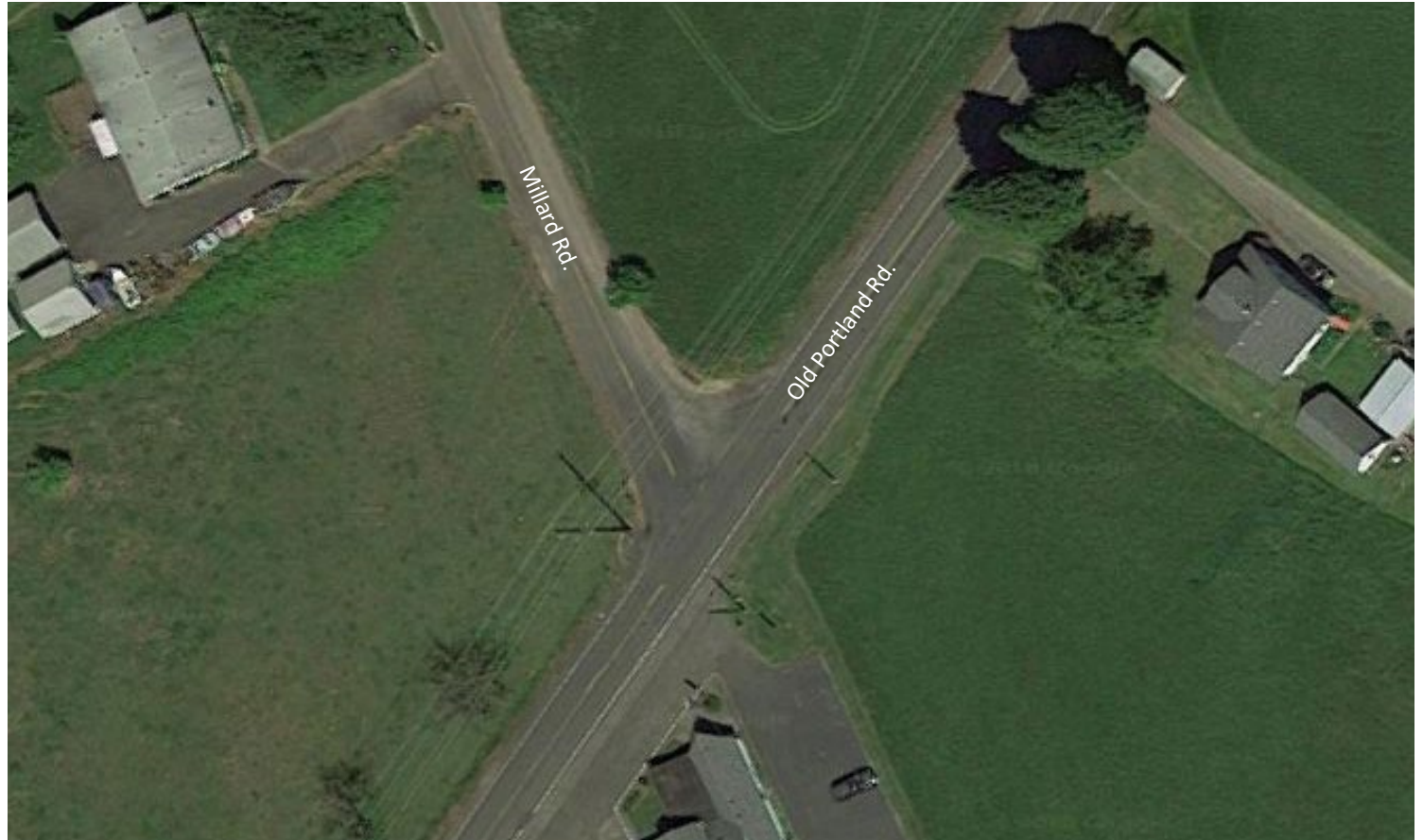
Existing conditions (image: Google Earth)
