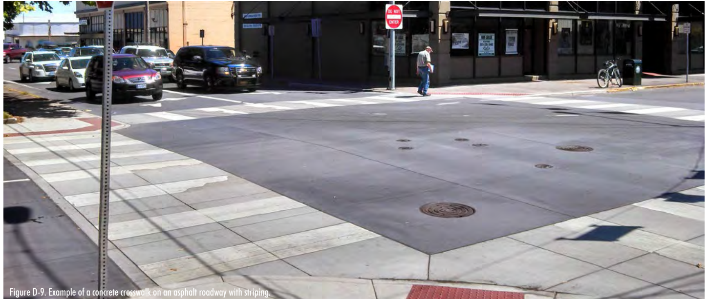
Figure D-9. Example of a concrete crosswalk on an asphalt roadway with striping.
