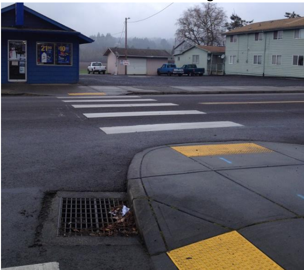
Crosswalk with bulbout at Market Street
