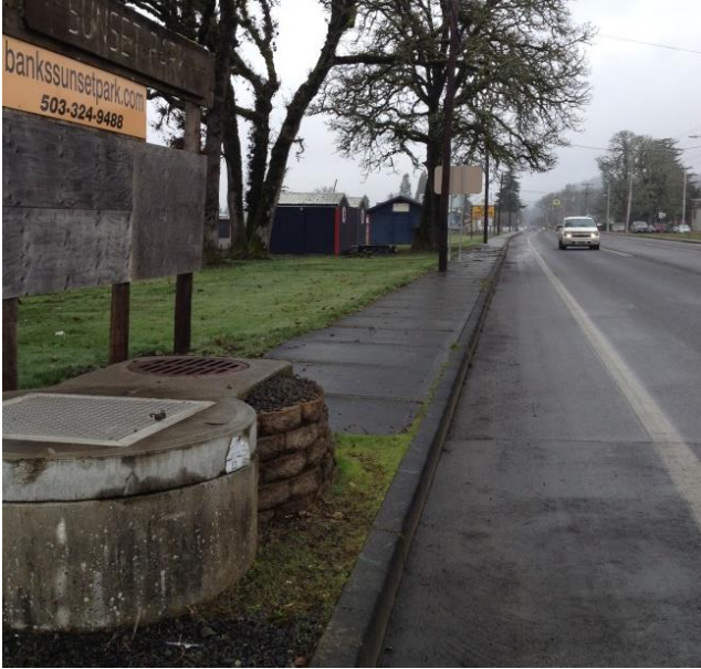
Sidewalk ending at Banks Sunset Park along Main Street (OR47)
