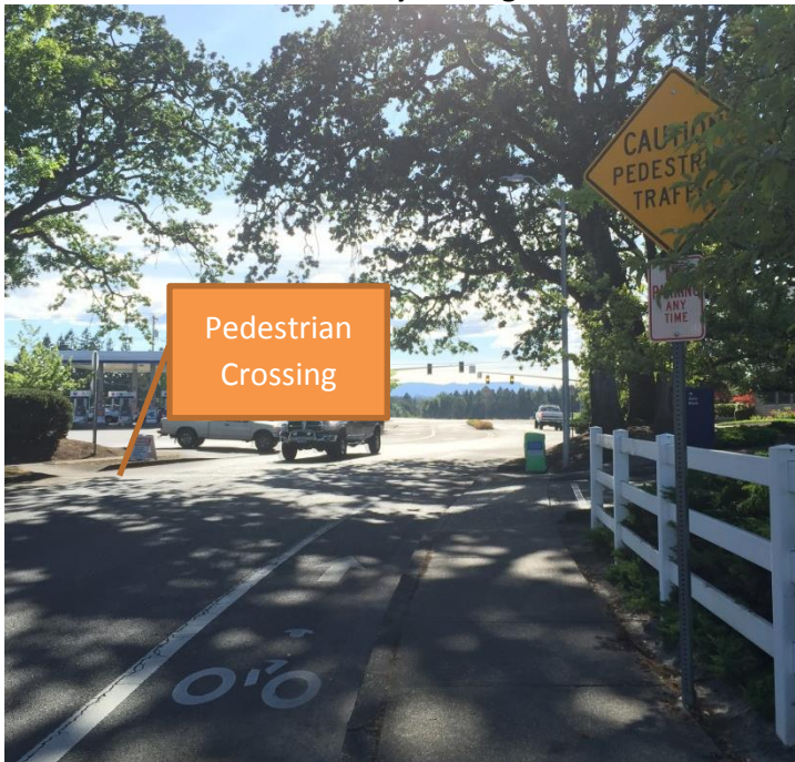
Exhibit 8-2 NW Oaks Way looking West
