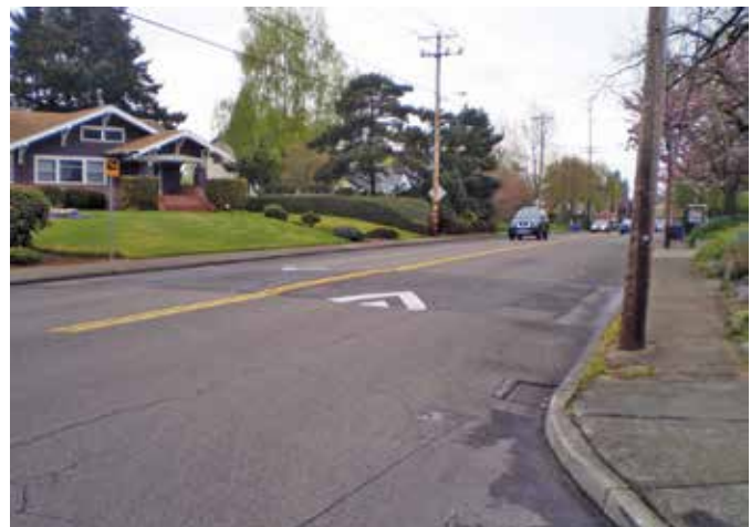
View of Roberts Avenue, classified in the TSP with “special street” cross-sections.
