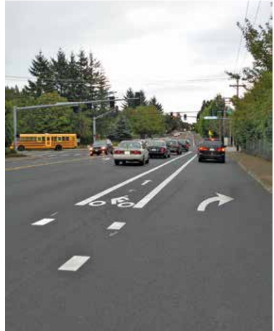
Right: Summer 2013 improvements on SE Powell Valley Road included a reconditioned street surface, revised roadway striping layout to add an additional west-bound travel lane and a new sidewalk connection between Gordon Russell Middle School and Burnside Road that completes a continuous walking connection from Burnside to Kane.
