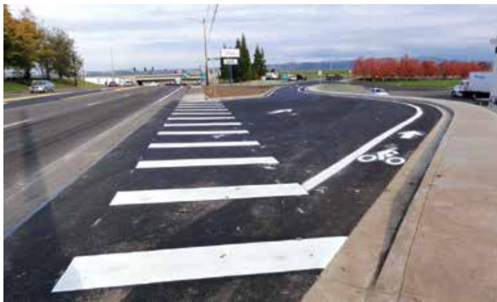
Freight improvements at NE 181st Avenue and Wilkes Road allow easier access to Interstate 84.
