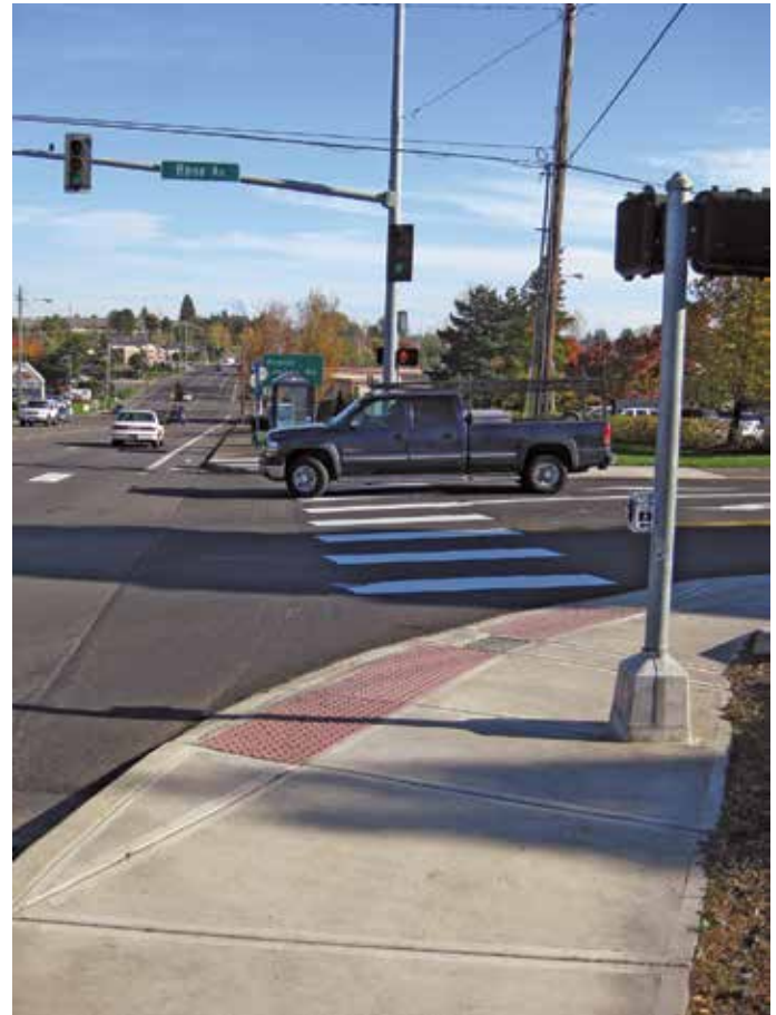
An ADA-compliant curb ramp on SE Rene Avenue.
