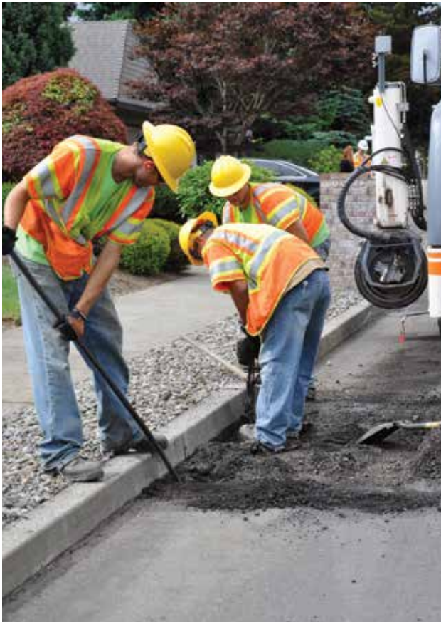
Left: City Transportation Operations crews repair a street's pavement.
