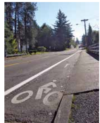
Bicycle lanes on SW Towle Avenue between the Springwater Trail and SW 10th Drive. Bicycle lanes are required on all streets except for those designated as minor collectors.
