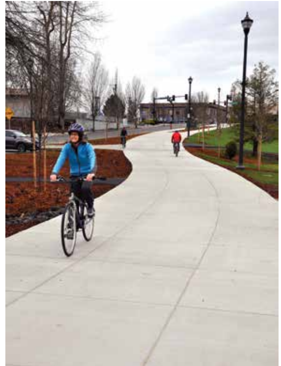
The new Springwater Spur Trailhead at Main City Park, completed in 2013, is part of the City's Bicycle System Plan to provide a system that continues to attract new cyclists to Gresham.
