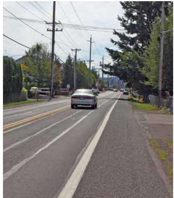
Missing sidewalk along NE Cleveland Avenue north of Burnside Road.
