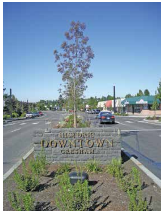
Traffic calming devices include planted medians, such as this one on Powell Boulevard.
