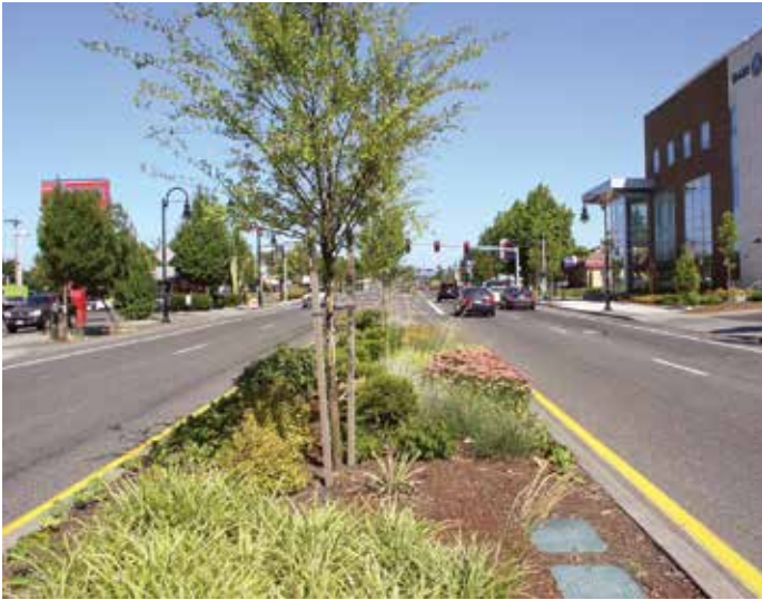
Access management used via planted median barriers on Stark Street west of 185th Avenue.
