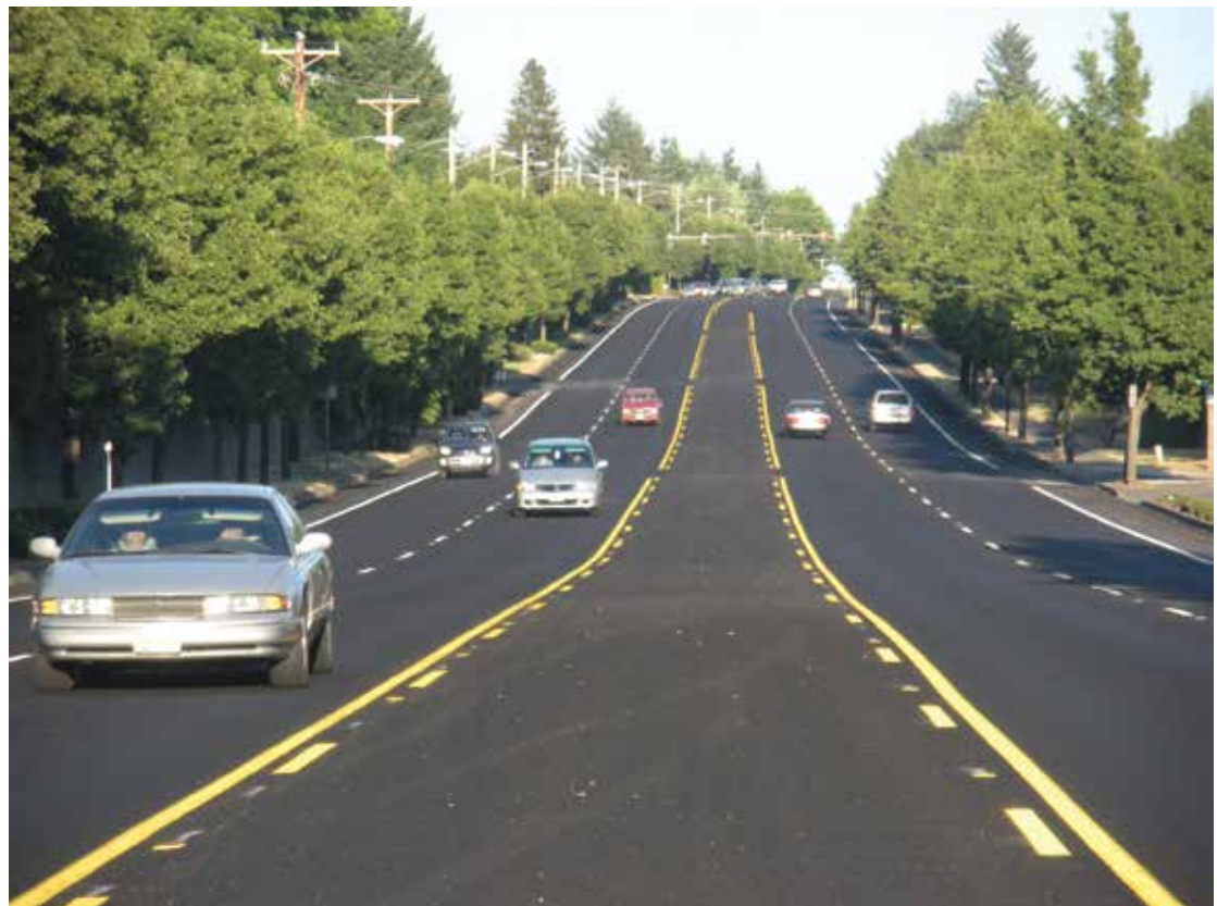
A segment of Burnside Road, a major arterial, after a microseal treatment.
