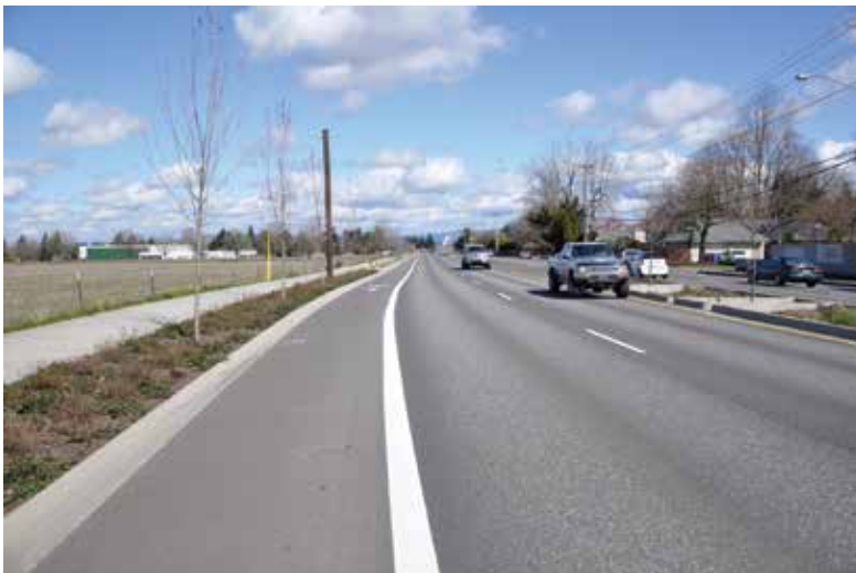
Hogan Drive - a major arterial - includes rain gardens, bike lanes, and planted medians.
