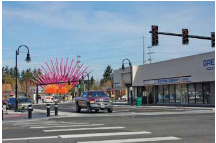
The area at SE 188th Avenue at SE Stark Street in Rockwood features underground utilities.
