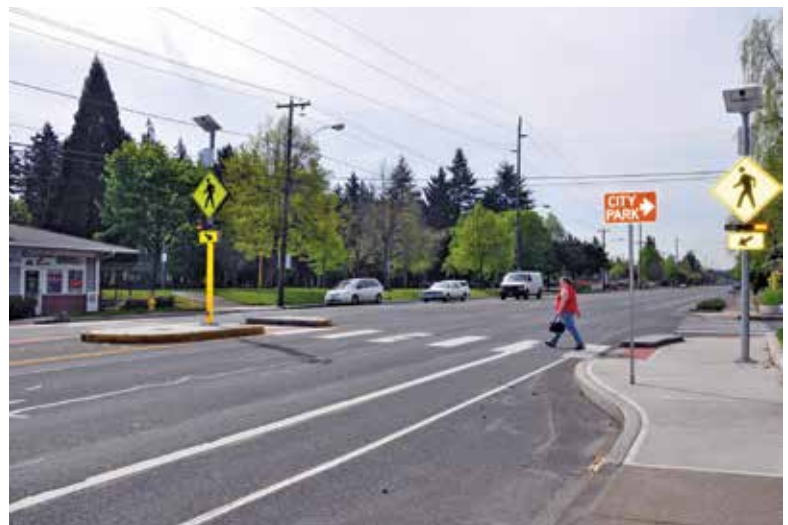
Raised medians benefit pedestrians by allowing them to cross only one direction of traffic at a time.
