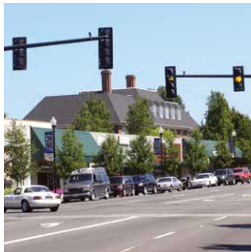
The intersection of E. Powell Boulevard at N. Main Avenue features flashing yellow arrow left-turn phasing.
