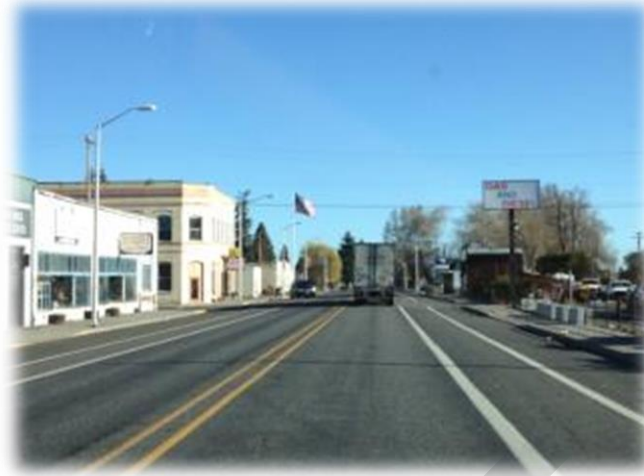
Exhibit 6-13. Existing Lighting in Grass Valley
