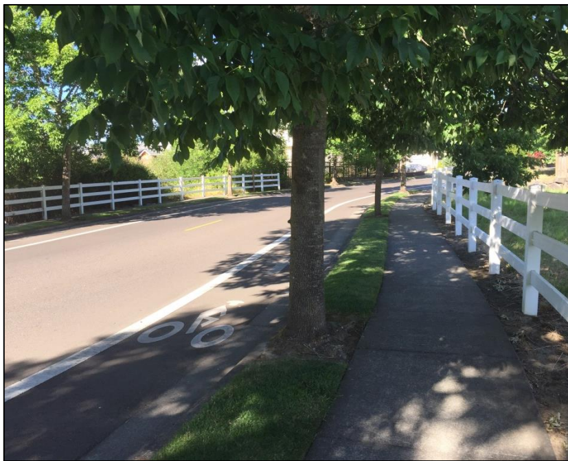
Westbound bicycle lane on NW Oak Way, landscape strip, and sidewalk
