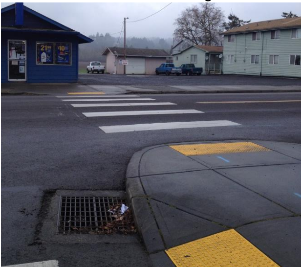
Crosswalk with bulbout at Market Street
