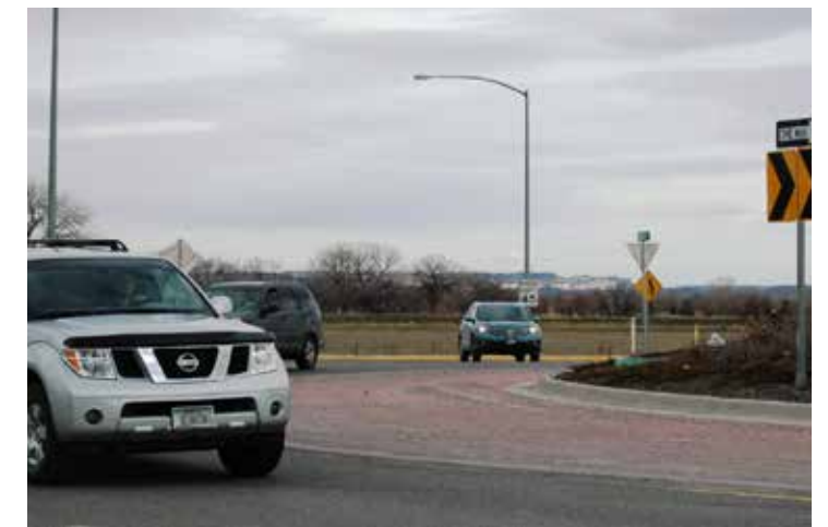
Exhibit 12.12 Roundabout on Shiloh Road
