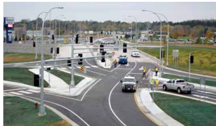
Exhibit 12.10 Diverging Diamond Interchange in Minnesota
