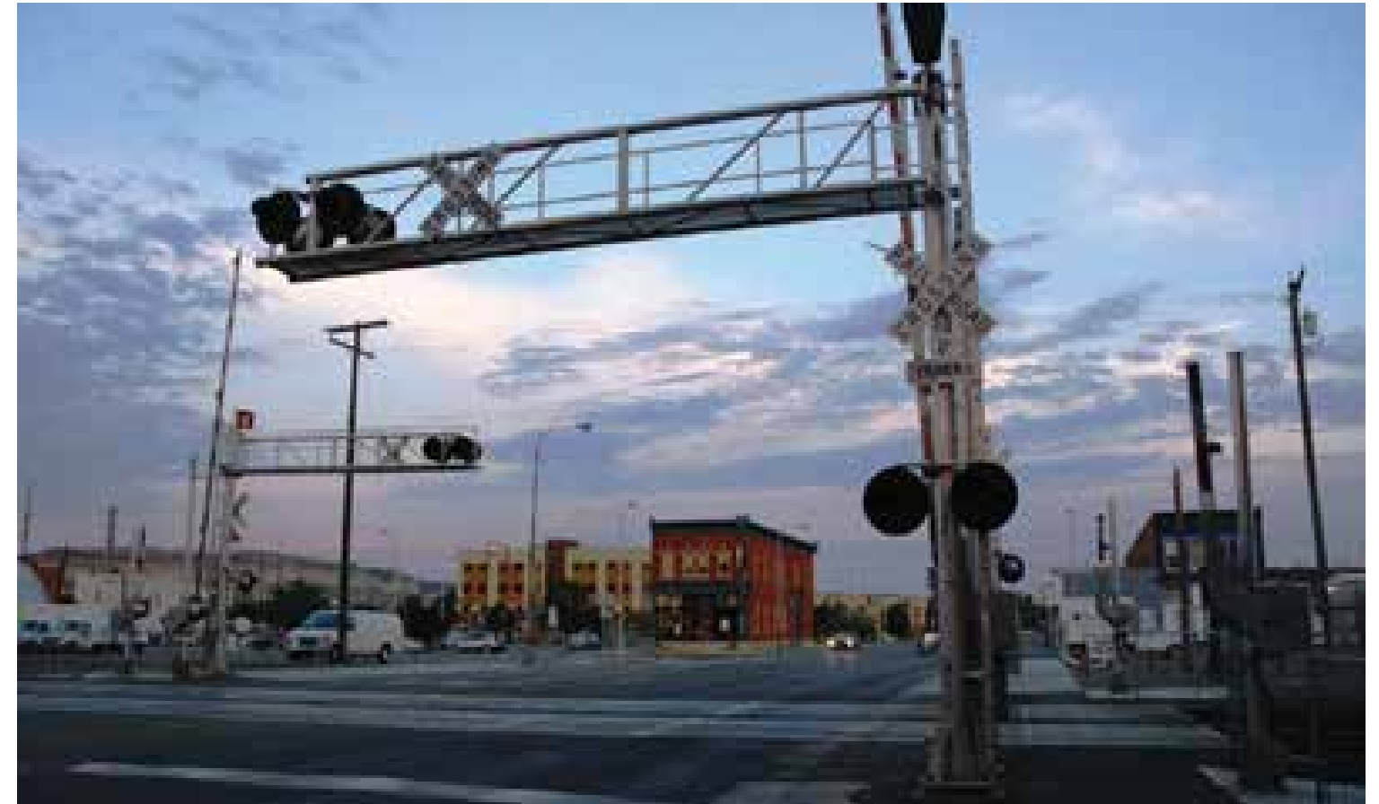
Exhibit 8.2 Rail and Pedestrian Crossing at 27th Street
