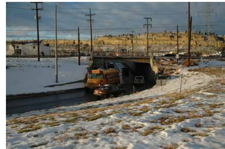
Exhibit 8.3 Rail Crossing at 13th Street
