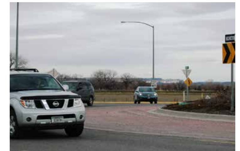
Exhibit 12.12 Roundabout on Shiloh Road
