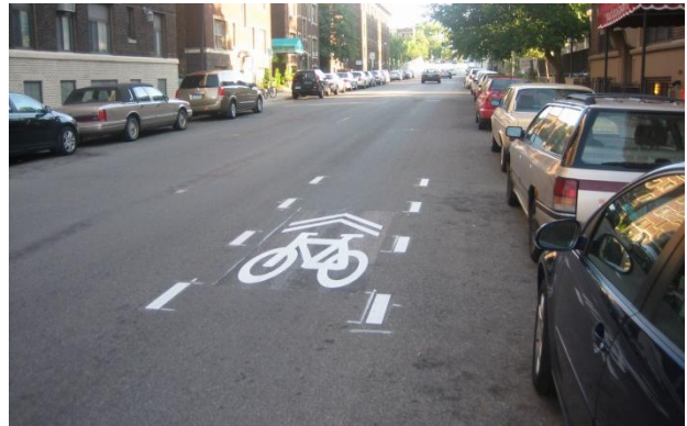
Example of a Priority Shared-lane Pavement Marking
