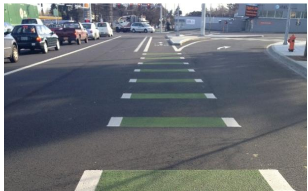
Example of Pavement Markings Through Intersection
