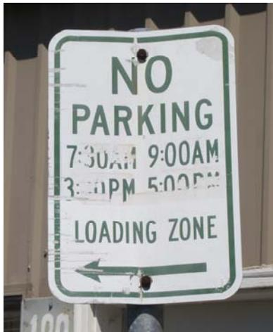
*This sign is located on Berkeley just west of Portland. It is in poor condition, and when it is replaced, it should have red legend on a white background.*
