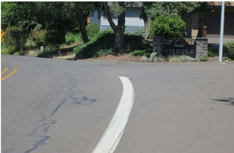
*We suggest that the City consider the installation of a series of Chevron signs on the outside of this curve to provide additional guidance to drivers.*
