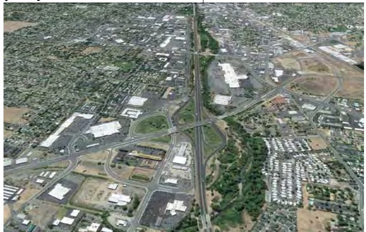
Interstate 5, center, at North Medford Interchange, looking south.
