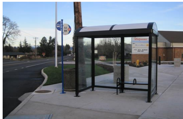
TriMet Stop (After)
