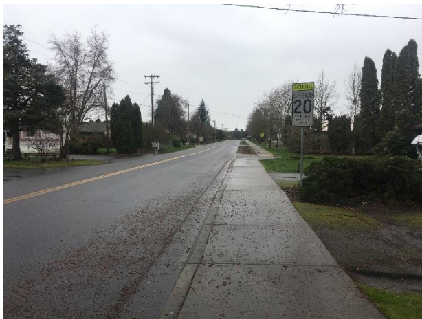
6-foot curb-tight sidewalk
