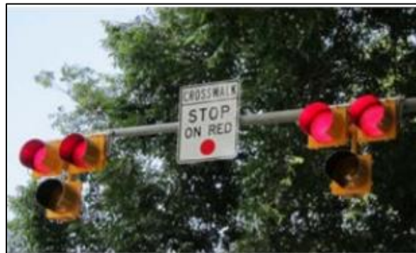
Figure 7 Example of a Pedestrian Hybrid Beacon Mounted on a Mast Arm [Source: (FHWA, 2015)].
