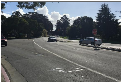
Figure 20 Location along Mission Road In Need of Traffic Control.
