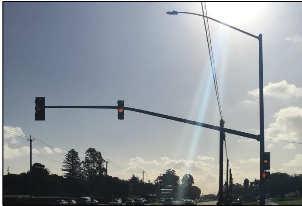
Figure 28 Limited Signal Visibility
