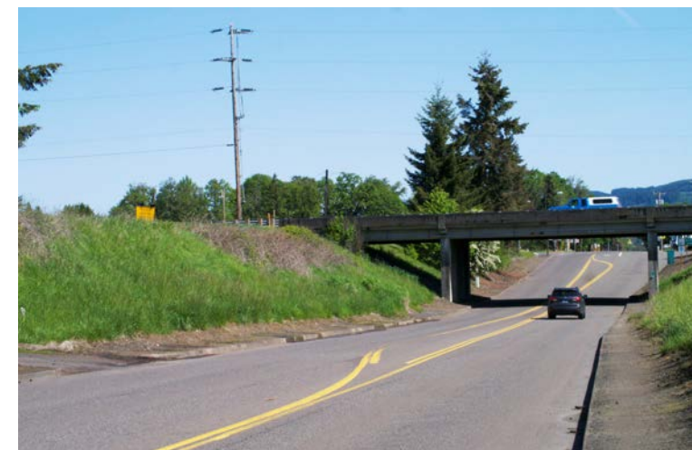
Oregon 6/Oregon 46 undercrossing looking north
