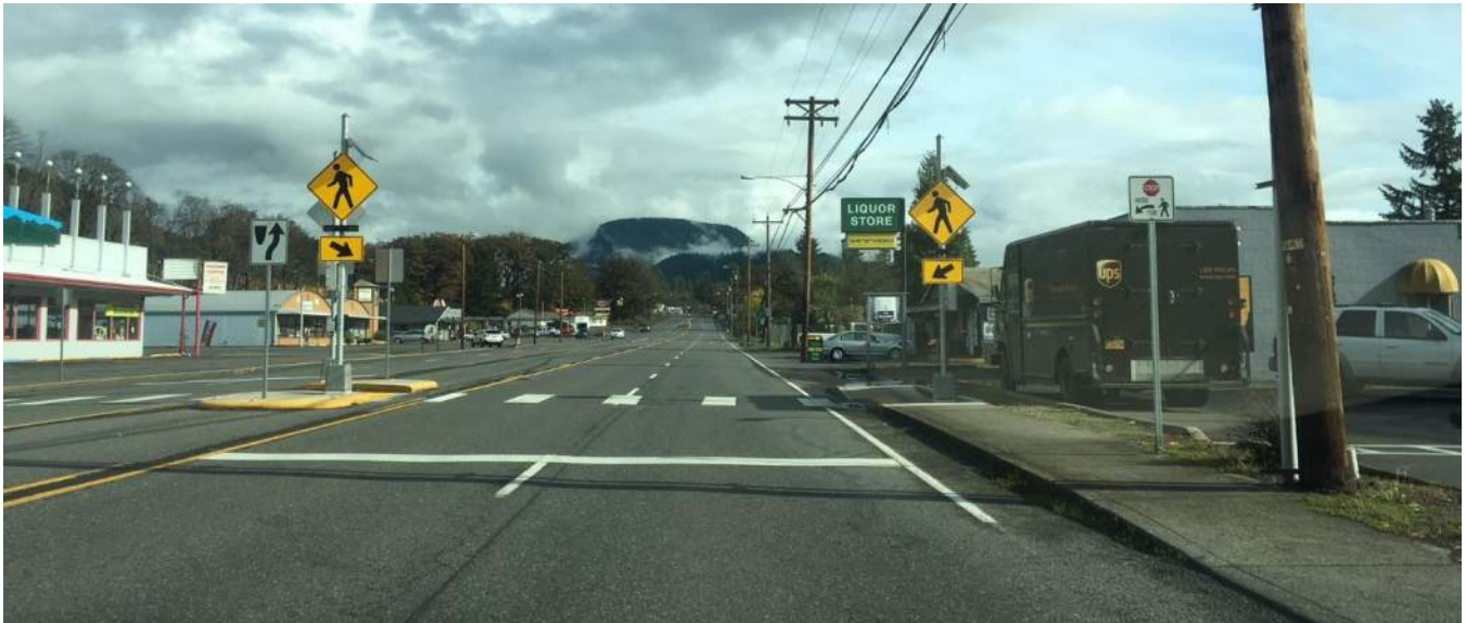
Illustration of Pedestrian Crossing with RRFBs Installed on OR 58, West of Rock Road
