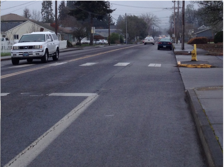
Bicycle lane ending at the high school entrance along Main Street (OR47)
