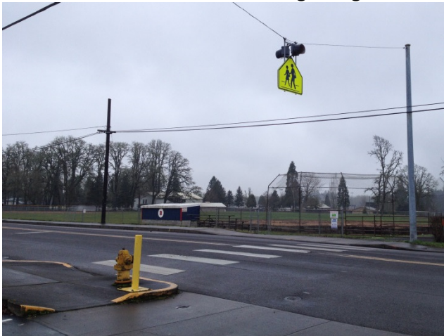
Overhead flashing pedestrian sign at the High School entrance along Main Street (OR47)
