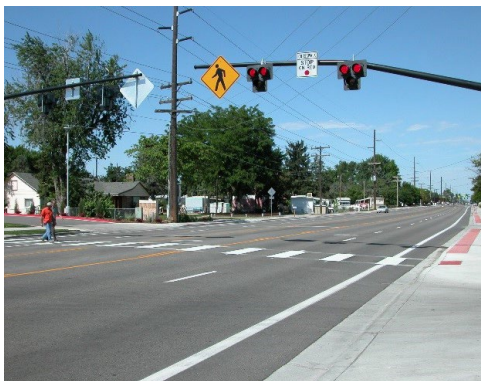
Crossing with Pedestrian Hybrid Beacon
