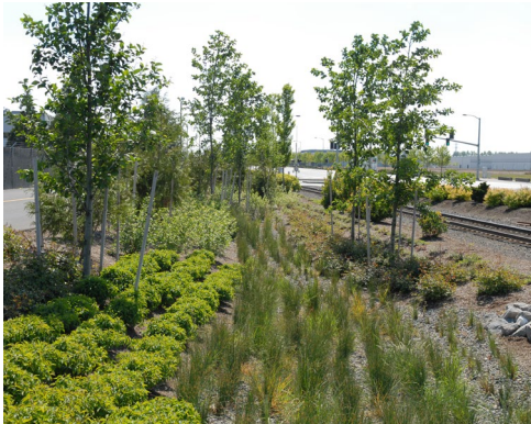
Large vegetated swale in north Portland, OR
