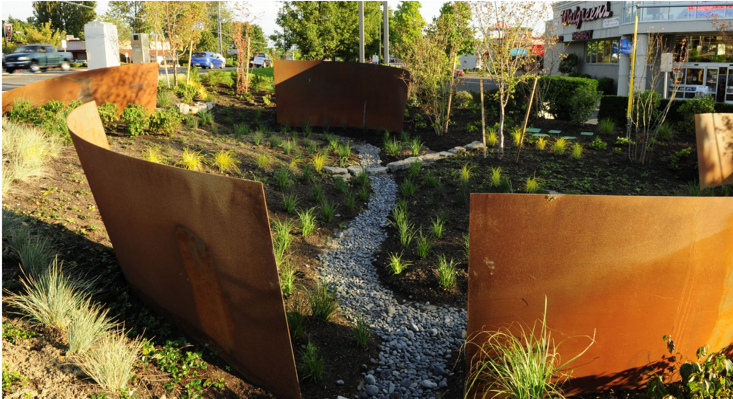
The Warner Milne Rain Garden in Oregon City collects stormwater and runoff from adjacent surfaces
