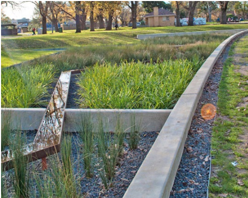
Artful rainwater conveyance in Melbourne, Australia
