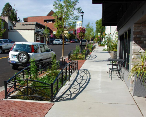
Stormwater planter with railing in Lake Oswego, OR
