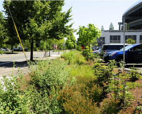
Mature stormwater planter along Water Avenue
