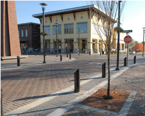
Change of materials at intersection in Washougal, WA
