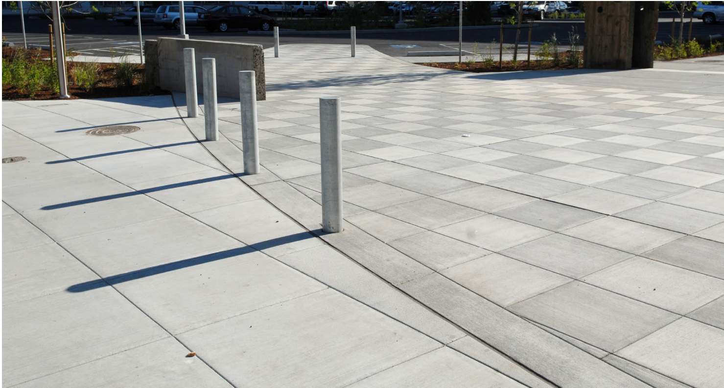
Scored concrete paving
