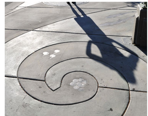
Decorative concrete paving
