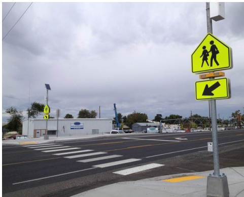
Crossing with Rectangular Rapid Flashing Beacon
