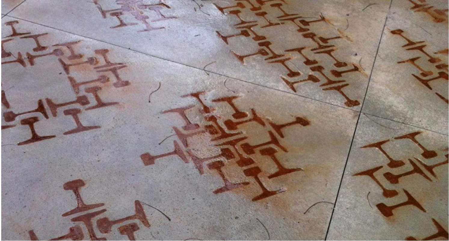
Stenciled concrete paving
