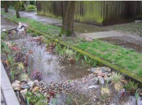
Swale retaining rainwater after a storm event
