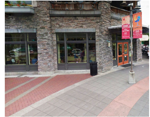
Brick and concrete paving
