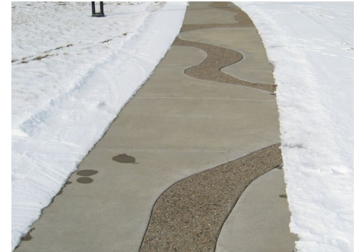
Concrete and aggregate paving
