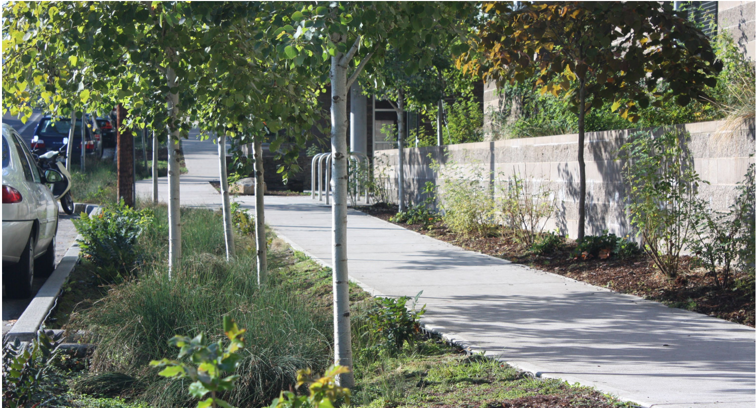
Trees and planting in a stormwater swale enhance the pedestrian experience in Portland, OR
