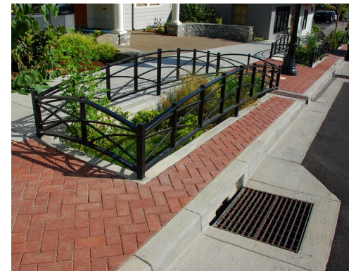
Brick and concrete paving
