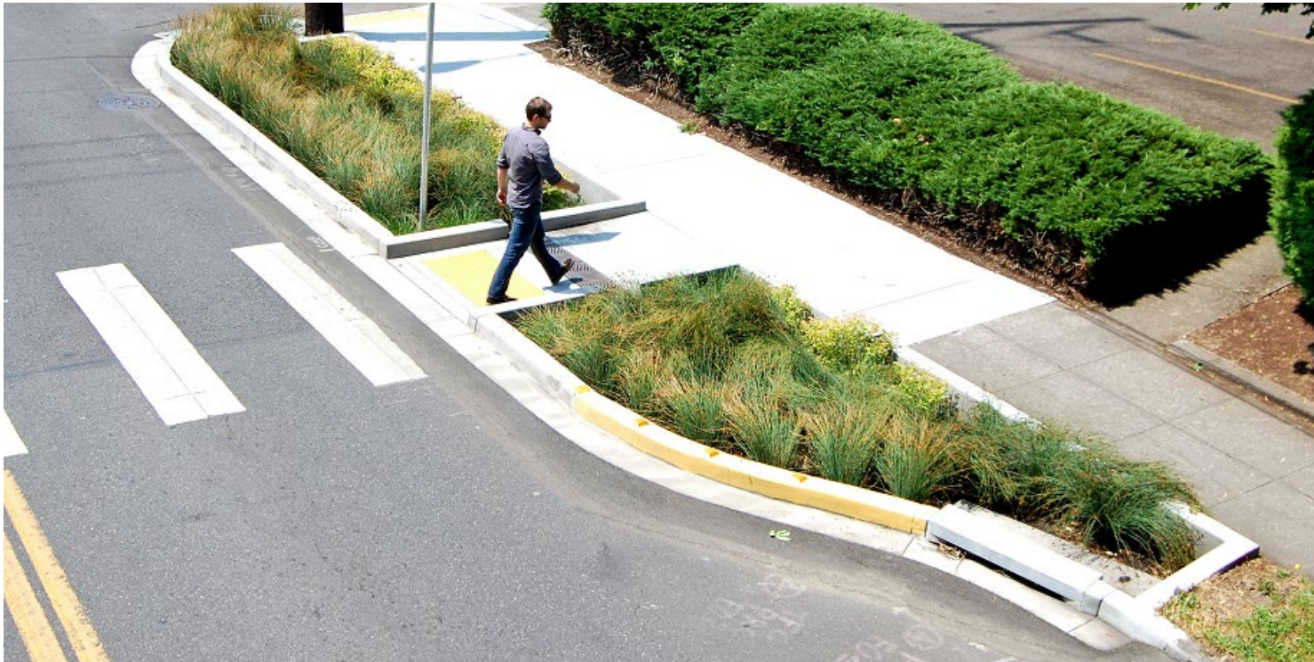
Bulb-out with stormwater facility and crosswalk
