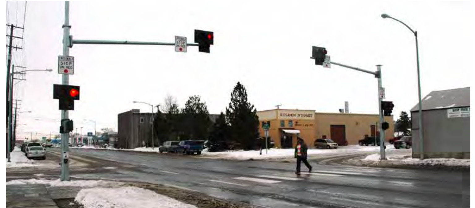
Exhibit 9.4 Pedestrian Hybrid Beacon (HAWK) at 4th Avenue in Downtown Billings
