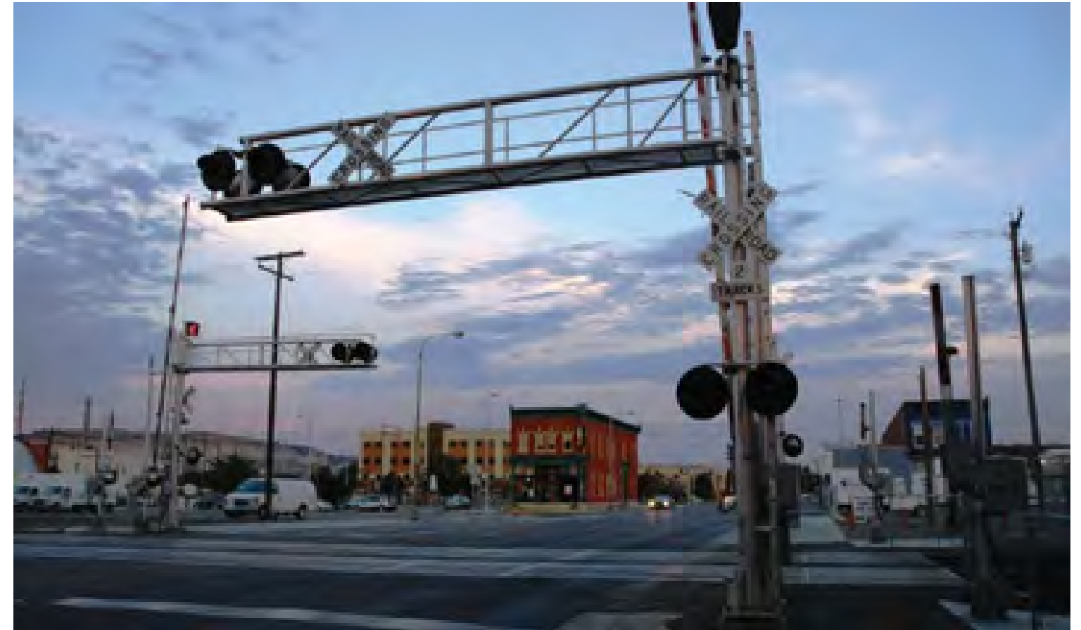
Exhibit 8.2 Rail and Pedestrian Crossing at 27th Street
