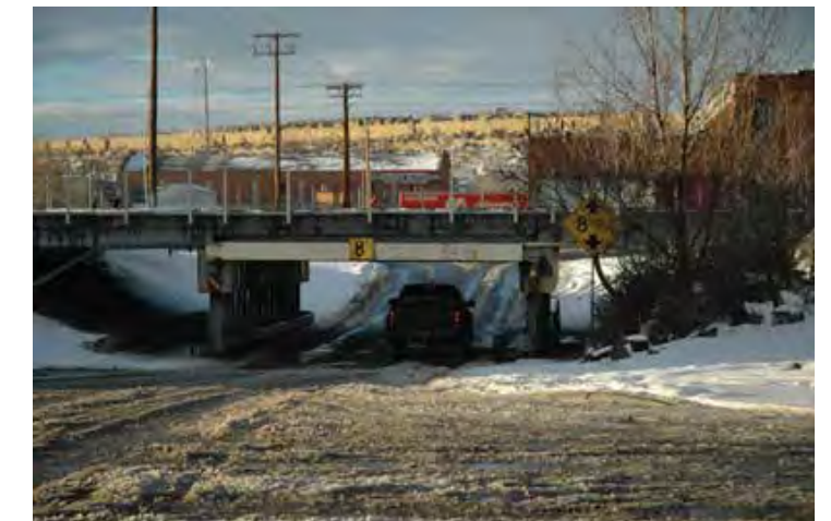
Exhibit 8.4 Rail Crossing at 21st Street
