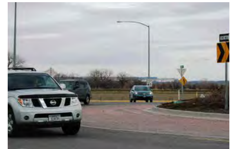
Exhibit 12.12 Roundabout on Shiloh Road
