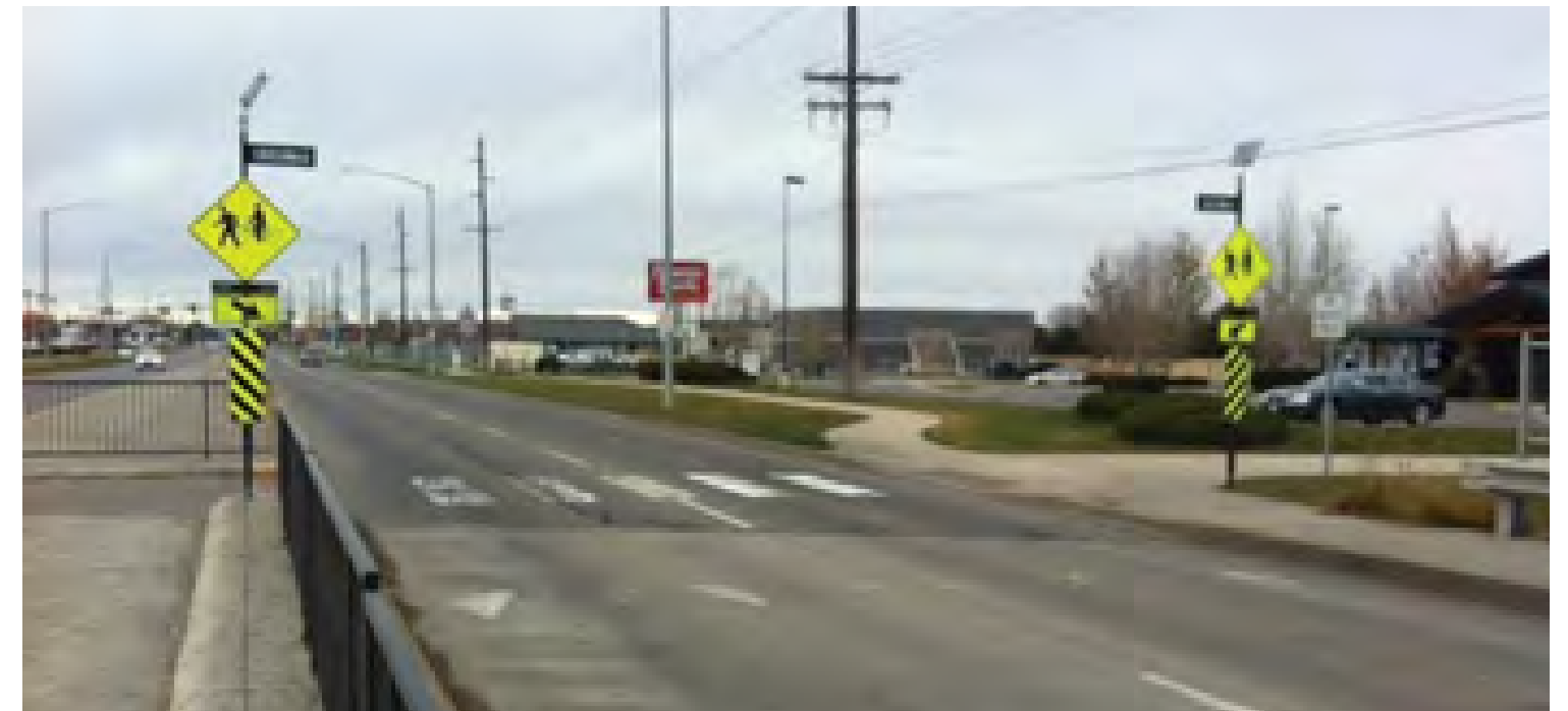
Exhibit 9.5 Rectangular Rapid Flashing Beacon (RRFB) on King Avenue
