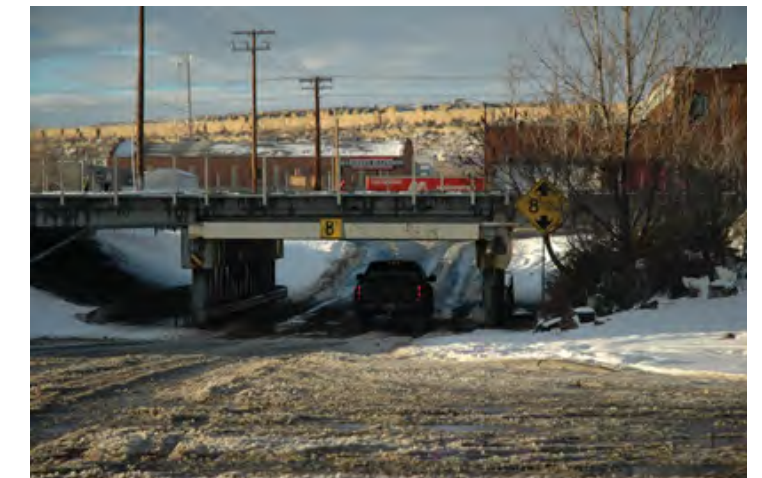
Exhibit 8.4 Rail Crossing at 21st Street
