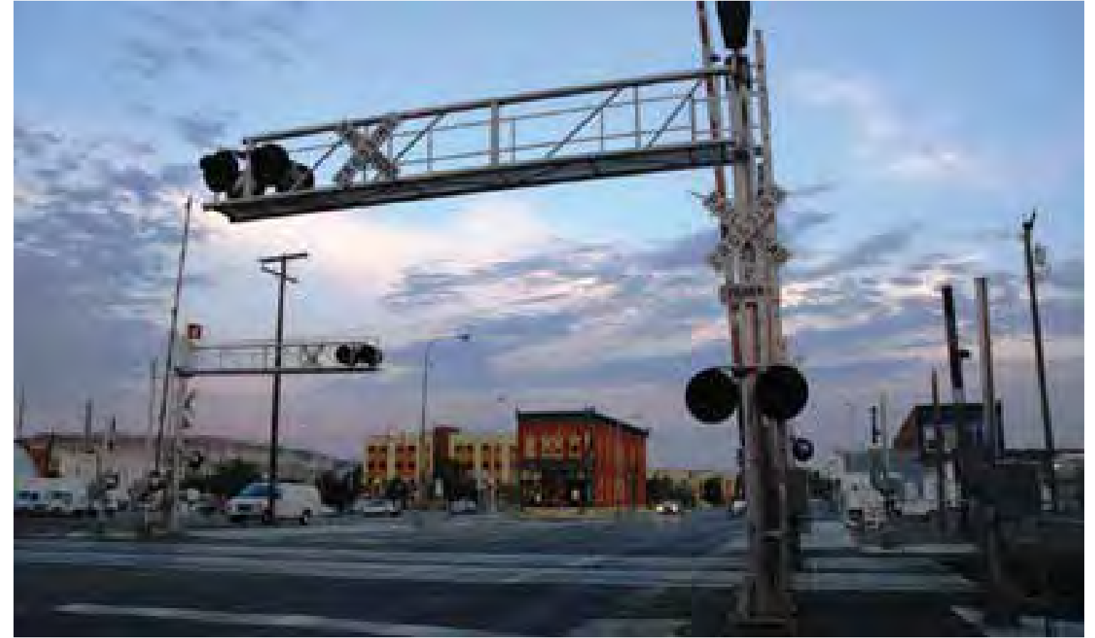
Exhibit 8.2 Rail and Pedestrian Crossing at 27th Street
