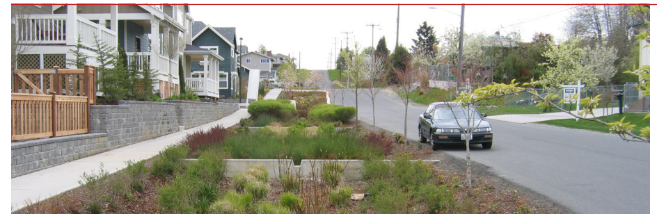
This is representative of the type of bioretention area that is recommended along the north side of C Street NE; however, the design will include walkways for providing access between the on-street parking and the sidewalk area.
