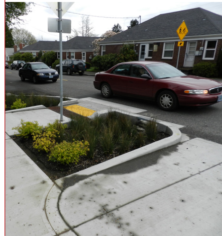
This is representative of the treatment that may be included at the intersection corners to capture stormwater runoff before it can reach the storm sewers.
