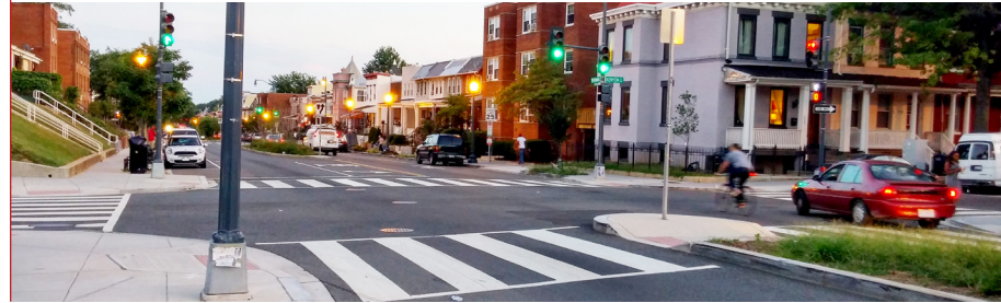
An example on Sherman Avenue NW where a curb extension and median refuge provides a shorter crossing distance and reduces exposure to moving traffic.
