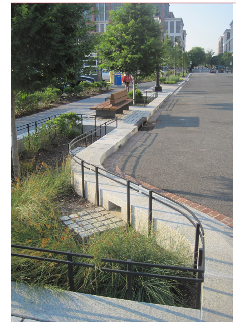
Low impact development at Navy Yard on 3rd Street SE.
