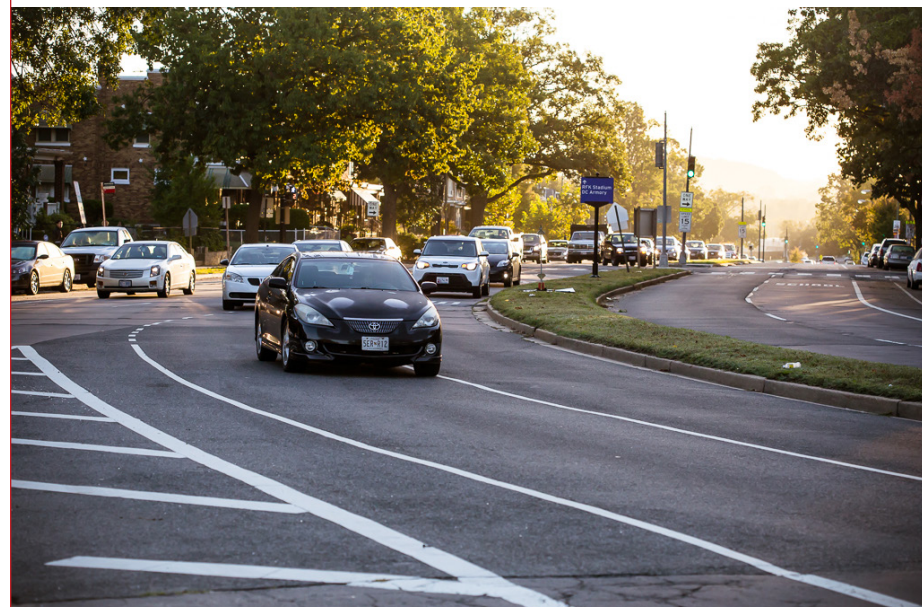
Traffic on C Street NE is very directional during the morning and afternoon periods, particularly the westbound direction during the morning peak period.
