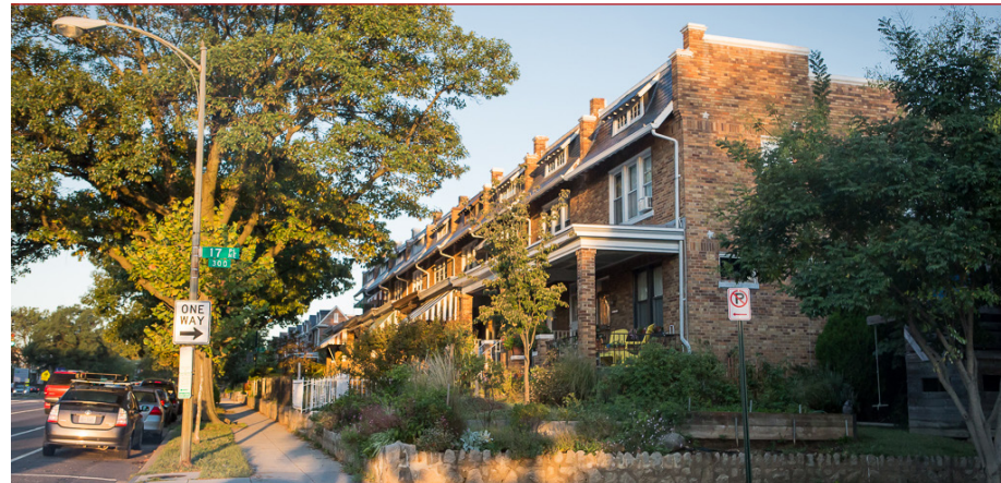
While C Street NE is designed to accommodate heavy commuter traffic, the area is predominantly residential.
