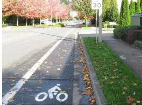
Curbed Roadway with Bike Lane and Sidewalk
