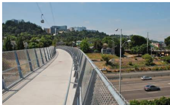
Pedestrian Over Crossing Portland, OR – I-5
