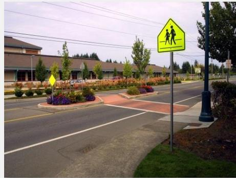
A raised median island provides a protected area in the middle of a crosswalk for pedestrians to stop while crossing the street. These refuges allow pedestrians to cross one direction of traffic at a time. Pedestrian refuges are often used in areas with high traffic volumes and/or at locations with a crash history involving pedestrians.
