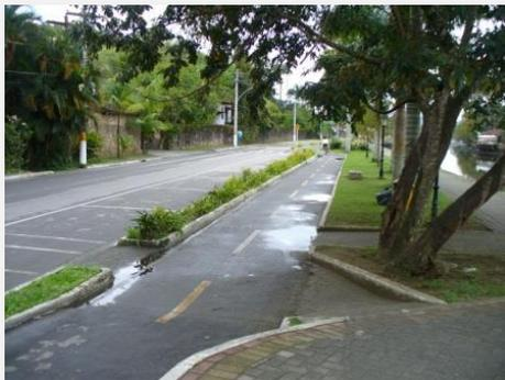
Cycletracks are exclusive bikeways separated from vehicle travel lanes, parking lanes and sidewalks. They can be one- or two-way in direction and can be even with the street, the sidewalk, or somewhere between. On existing streets, cycletracks can be constructed where there is sufficient roadway width and/or in contexts where the number of vehicular travel lanes can be reduced.
