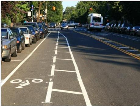
Buffered bike lanes are on-street bike lanes that include a physical separation (“buffer”) between the bike lane and the vehicle traffic lane and/or the vehicle parking lane. Buffered bike lanes can be particularly helpful on streets with high vehicle speeds, high vehicle volumes, or relatively frequent parking turnover.
