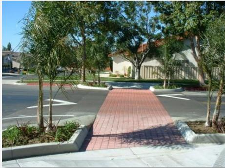
A raised crosswalk is raised higher than the surface of the street to give motorists and pedestrians a better view of the crossing area. A raised crosswalk is similar to a speed table and are often marked and signed for pedestrian crossing. Raised crosswalks are often used in areas with low speeds where people and difficulty crossing the street.
