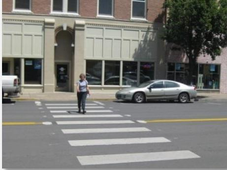
Clear, reflective roadway markings and accompanying devices are placed at intersections and priority pedestrian crossings where there is sufficient sight distance and reaction time for motorists to yield. Crosswalks can be used at intersections and at mid-block crossings.
