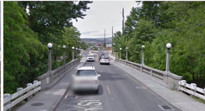
West 6 th Street Bridge
